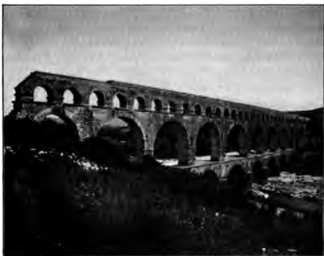
AQUEDUCT AT NÎMES, FRANCE, built by Antoninus Pius to supply the city with water from distant mountain springs; present condition of the structure where it crosses a deep valley.
